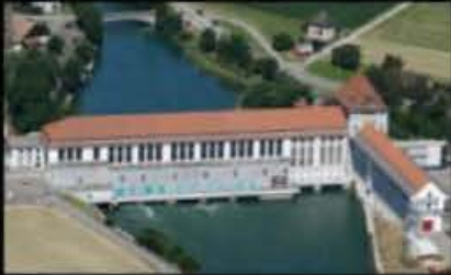
Hydroelectric power plant Residual/renewal energy for H 2 production
