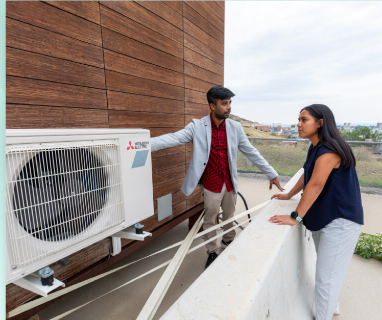
Photo by Werner Slocum / NREL
