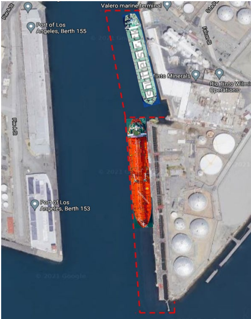
Figure 7-13 Illustration of the property boundary line of terminals (The figure is used only for illustration purposes. The measurement is not accurate.)
