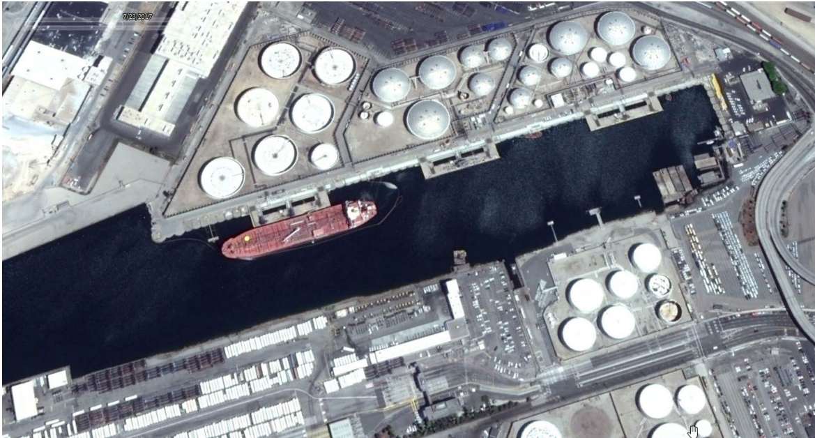
Figure 6-11 Satellite photo of a tanker berthing on the starboard side at Marathon Long Beach Berth 78
