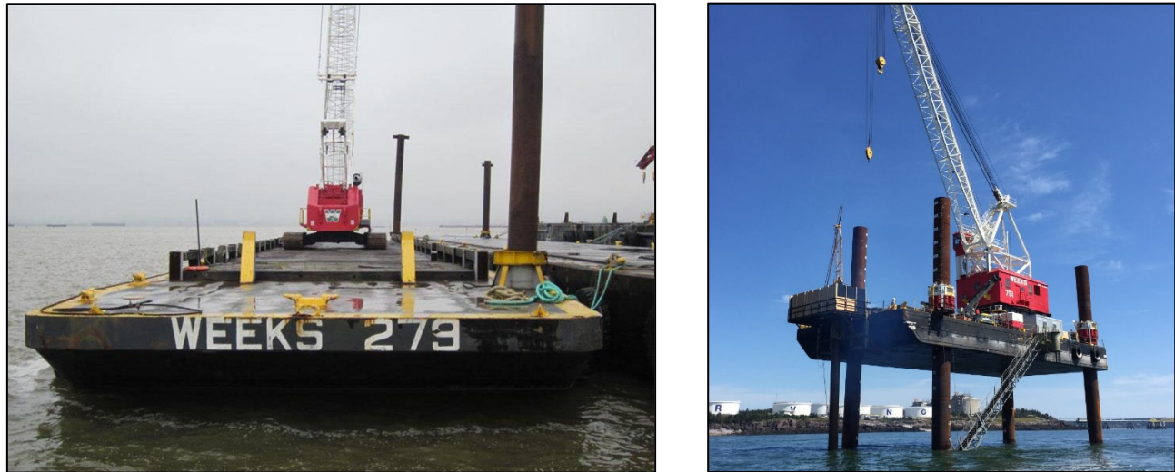
Figure 8: Spud Barge (left) and Jack-up Barge (Right) (Source: Weeks Marine)
