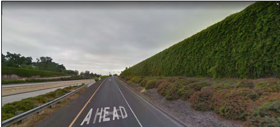
Figure 4-34-4 Vegetative Barrier w/ Solid Barrier on Highway 198, Visalia, CA
