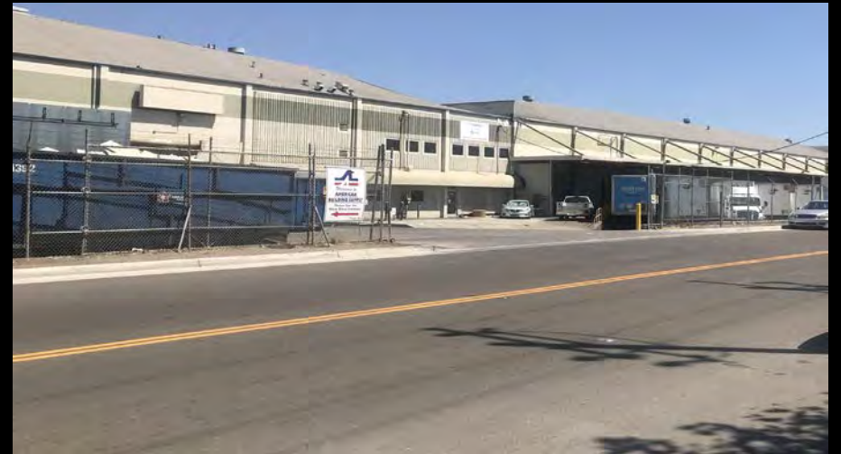
American Building Supply Inc.
