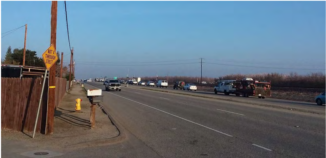
Figure 4 - Existing Highway 43 Shoulder Looking North
