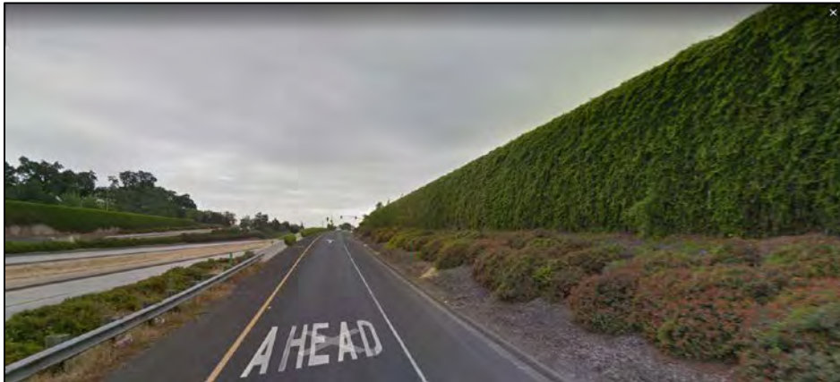
Figure 4-7 Vegetative Barrier w/ Solid Barrier on Highway 198, Visalia, CA
