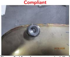
Figure 3. After the set screw is drilled out to make the new configuration tamper-resistant
