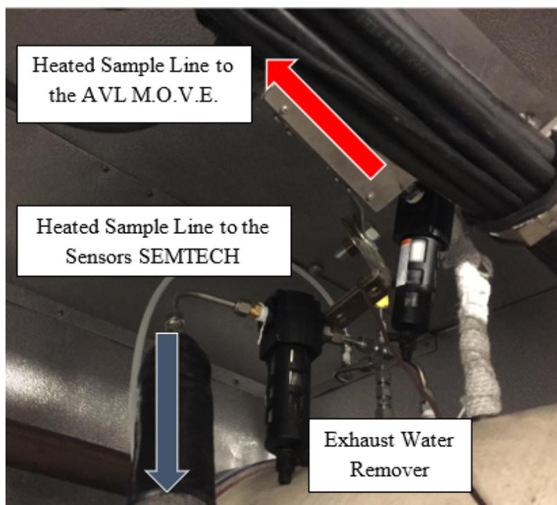
**Gas and PM exhaust ports on Vessel A. Exhaust water removers are installed before the heated sample lines.**
