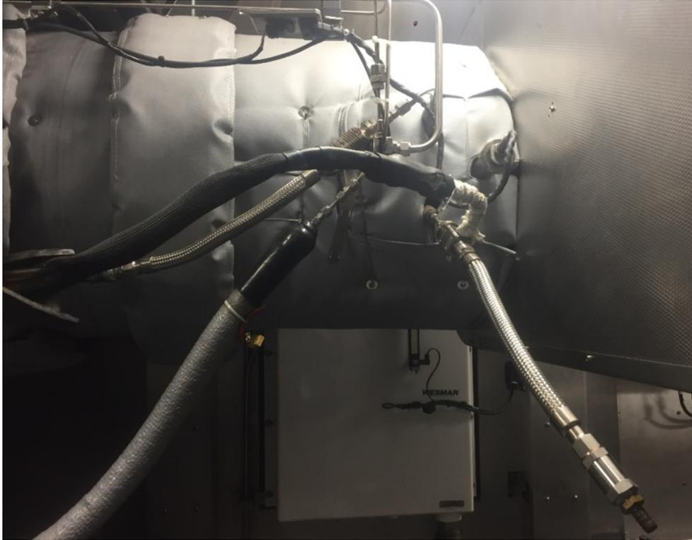
**Pre-SCR sampling position in the engine room of Vessel B.**
