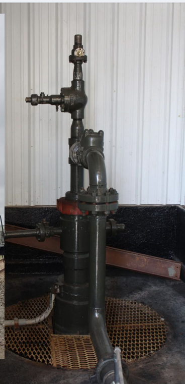
Injection Site, January 2021
