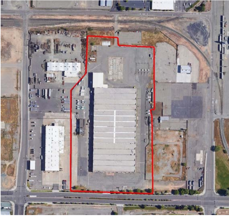
Figure 4-4 McClellan Garage - Existing Conditions | Source: WSP
