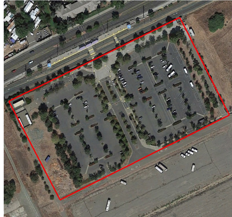
Figure 4-5 Hazel Garage - Existing Conditions
