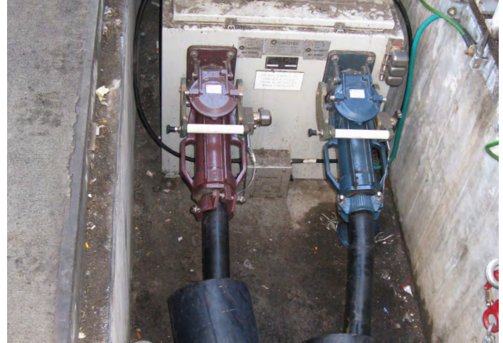
A shore power vault connection.
