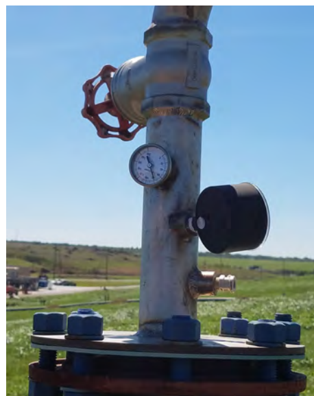
A landfill wellhead for maintaining methane gas flow.
