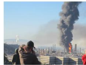
2012 Chevron Richmond Explosion
