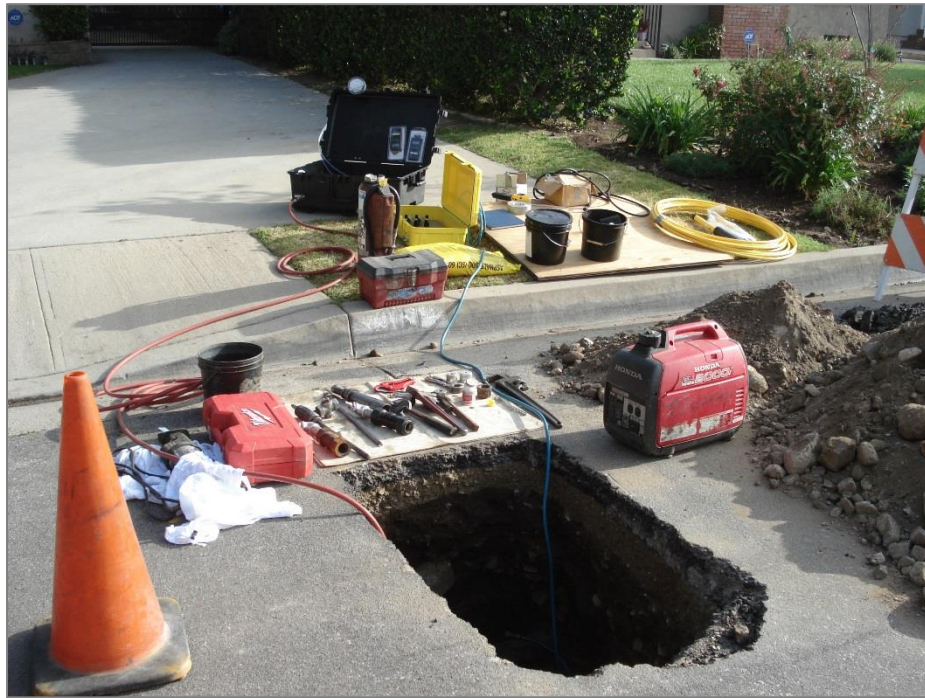
Figure 31 – Bell hole excavation for belowground leak measurements
