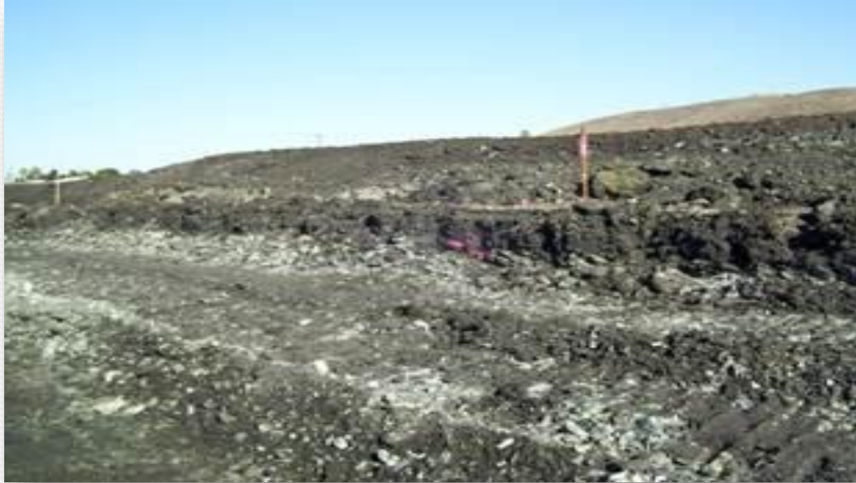
Photograph showing suspect serpentine NOA soil being excavated prior to analysis.
