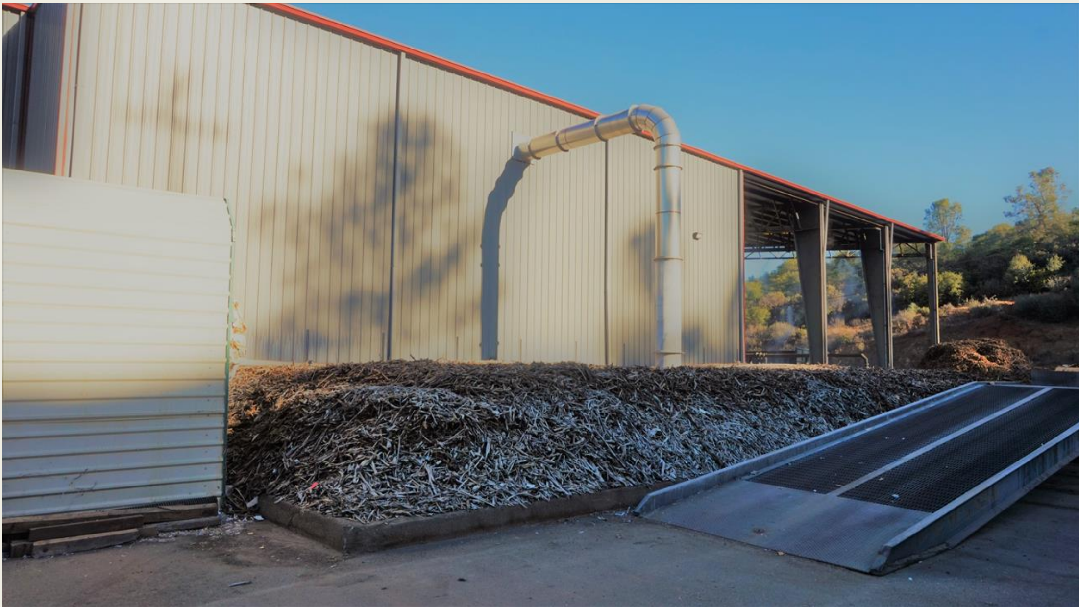
Biofiltration of the air to scrub odors
