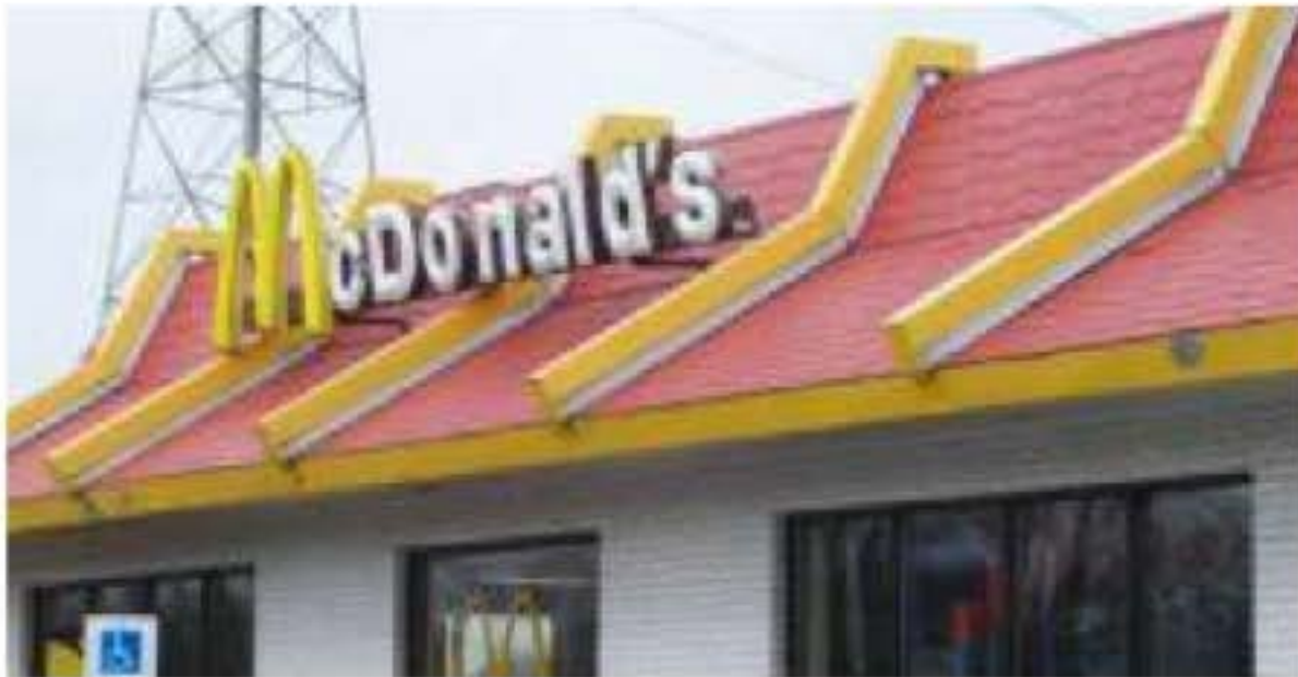
2 layers of 10% chrysotile shingles
