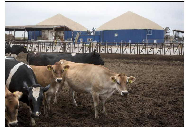
Methane digester on California dairy farm. Source: Andy Alfaro – aalfaro@modbee.com
