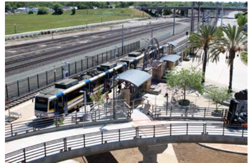
Bike and Pedestrian Bridge over Union Pacific Railroad
