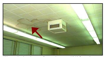
Water leaks in roofs and near HVAC units are common causes of moisture and mold problems.
