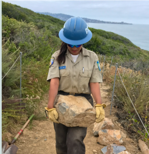
Figure 13. Young people employed through the California Conservation Corps work on projects from dead tree removal and forest health management to tree planting, trail building, and floodplain and riparian restoration. They receive on-the-job training as well as structured career guidance.
