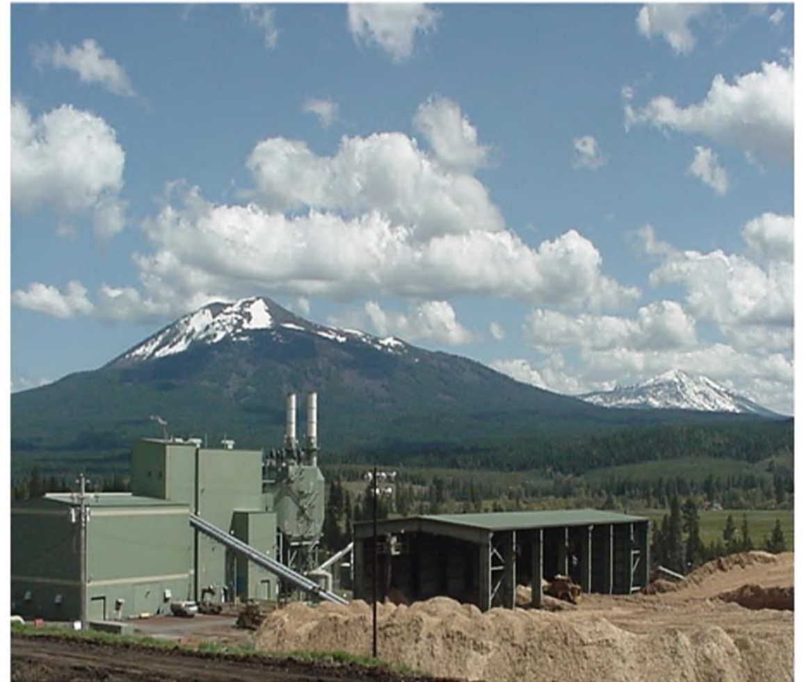
Controlled Combustion in a Biomass Powerplant Boiler
