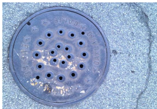
Sewer manhole cover manufactured and installed in Oakland, California
