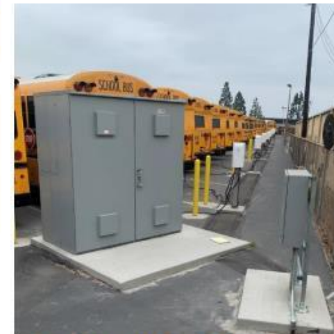
Switchgear, Nuvve Chargers, and Blue Bird RE Electric Buses
