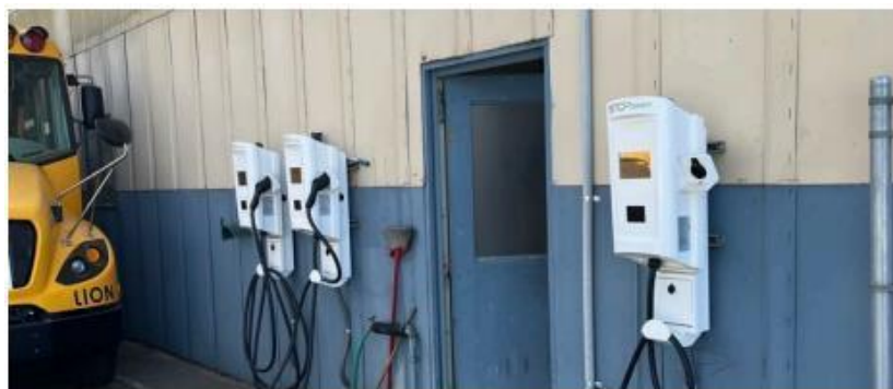
Charging installation at the site depot showing L2 chargers, above-ground conduit run, and switchgear
