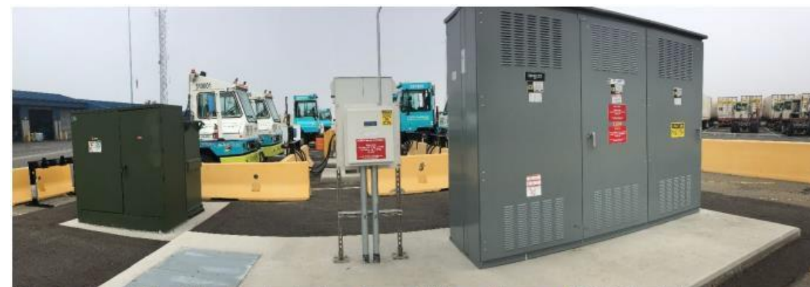
Charging installation at the site showing transformer (left), one three-port DCFC (center), switchgear (right), and several yard tractors (rear).
