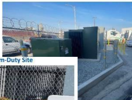
Figure 115. Final Deployment of Transformer and Switchgear Pad and Island
