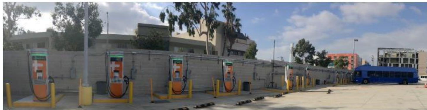
Charging installation showing chargers, above-ground conduit run, and a bus charging
