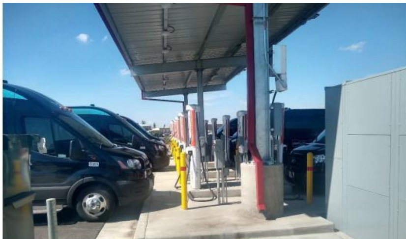
Charging installation at the site depot, showing chargers and multiple shuttle vans charging
