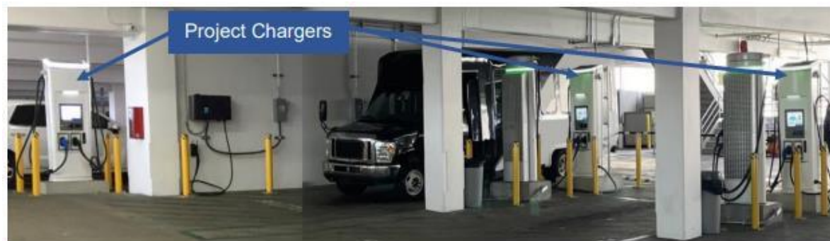
Existing ChargePoint CPE-250 Chargers, Delta Electronic Wallbox (center), BTC Power DCFC (left), and Endera/Lightning eMotors Electric MD Transit Buses
