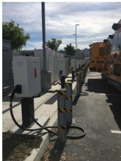
Site Layout Showing Nine of 12 Power Electronics Dispensers (small units) and Power Cabinets for 60 kW Rotational Charging (white boxes at image center)
