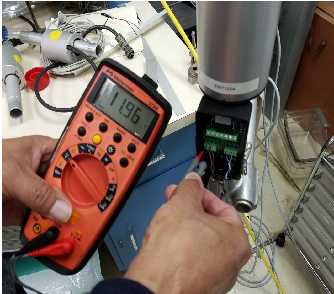
Figure 5: Checking 3D Sonic Input Voltage
