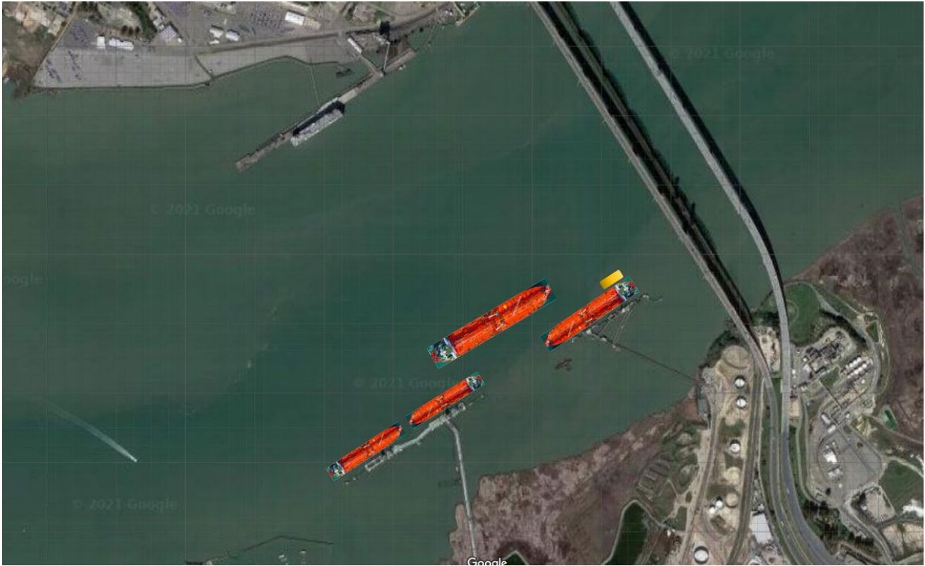
Figure 7-12 Illustration of the potential impact on the traffic at Carquinez Strait from the usage of barge-based capture and control technology (The figure is used only for illustration purposes. The measurement is not accurate.)
