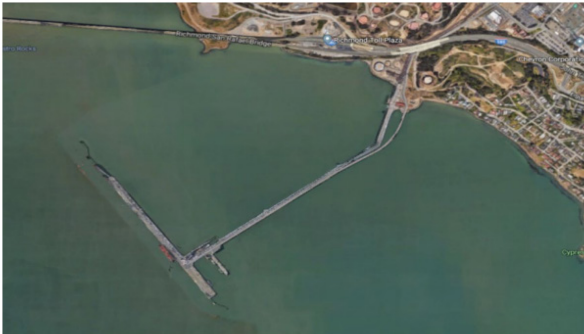
FIGURE 4: “T”-SHAPED MARINE OIL TERMINAL IN NORTHERN CALIFORNIA 47
