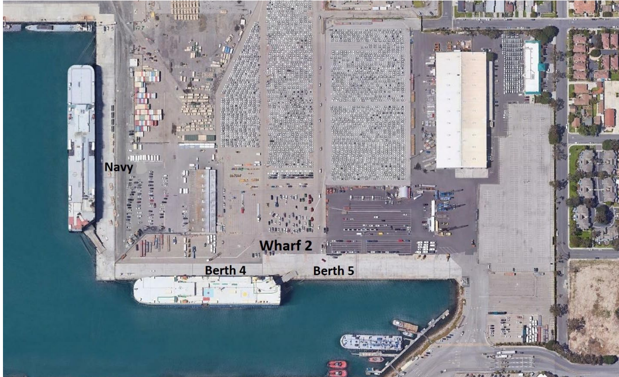
Figure 3-1: Port of Hueneme North Terminal (Wharf 2)
