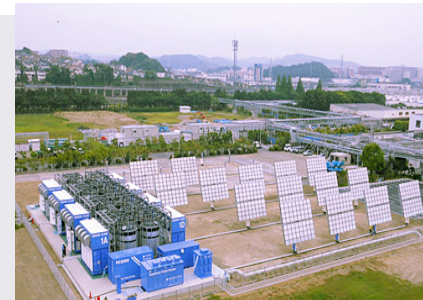
Integrated 1 MW solar photovoltaic and battery storage system
