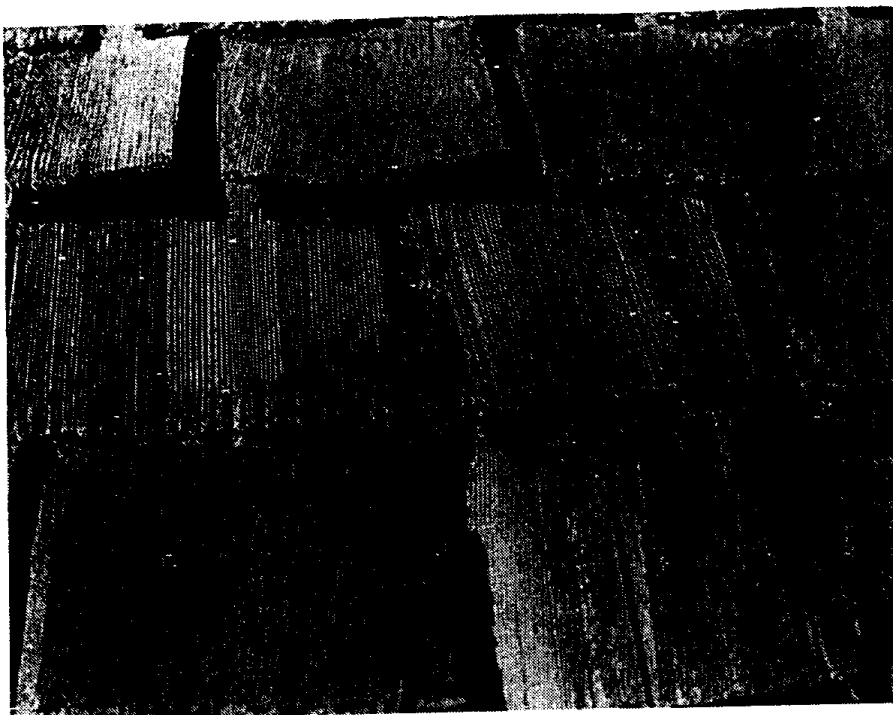
These 12 year-old shingles from an arid climate suffer more from sunlight than wood decay: the UV breaks down the wood, leading to cupping, curling, and splitting. Oil-borne treatments are needed to fight these drying stresses.
