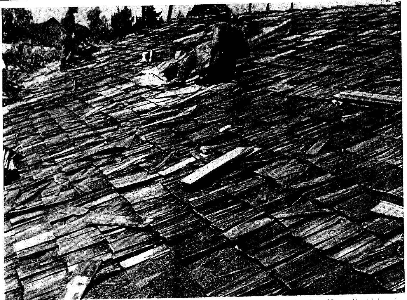
Any wood roof that requires more than 30 repairs per square, such as this one, is probably not worth restoring. Shingle roofs over 20 years old and shake roofs over 30 may be too far gone.
