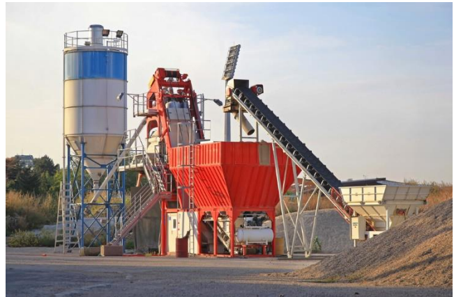
Figure 5f-1: Concrete batch plant
