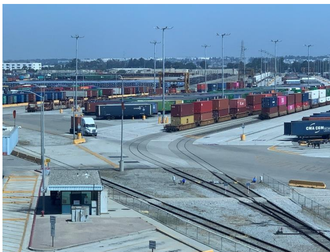
Figure 5f-1: Union Pacific Intermodal Container Transfer Facility (ICTF)/Dolores
